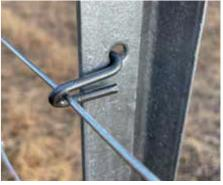
Locked In: The Rapid Clip appears loose once in but the narrow hook over the line wire prevents from rotating and coming out of the post hole
