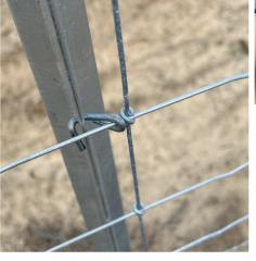
**Locked In:** The Rapid Clip appears loose once in but the narrow hook over the line wire prevents from rotating and coming out of the post hole
